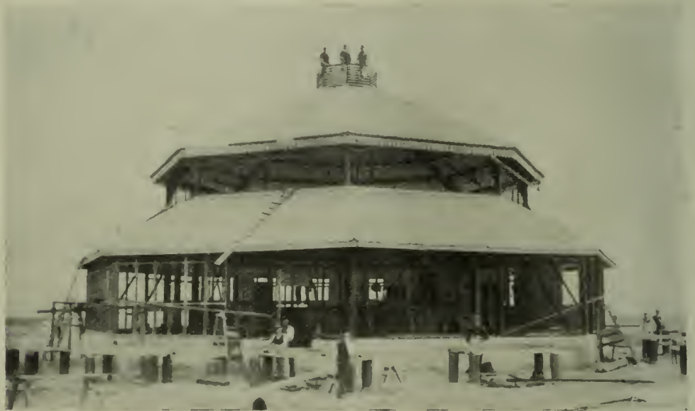
FIG. 2. THE FISH MARKET IN COURSE OF CONSTRUCTION.
